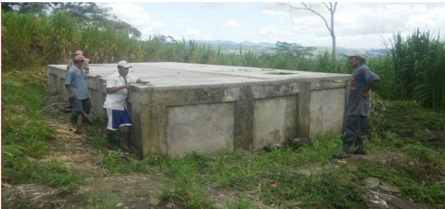
Community members participate in the construction of a water storage tank.
