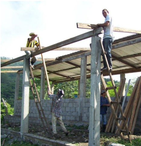
A new stable for the community's dairy cows is scheduled for completion in the next quarter.
